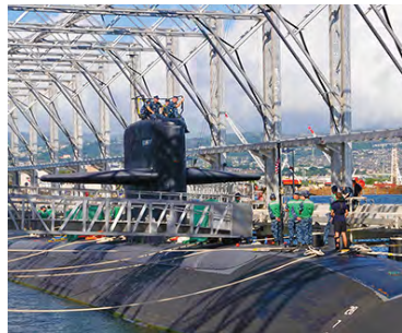
2002 Planning and design of the Pearl Harbor Magnetic Silencing Facility concrete slip.
