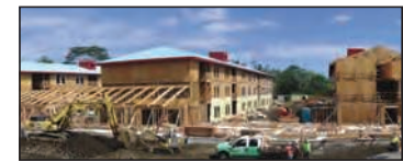
Construction in progress
