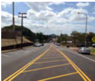
Ulune Road complete street demonstration project.
