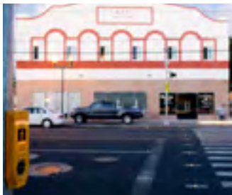
North King Street pedestrian safety pilot project flashing beacon and in-ground lights.
